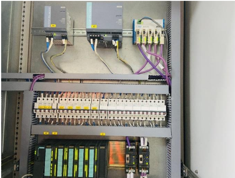
Figure-3: Five (5) channel repeater installed in the packaging line
